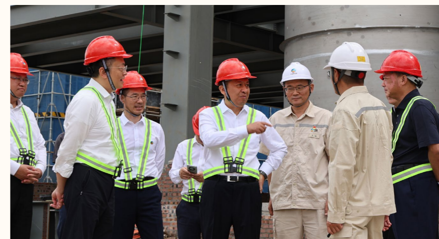
中粮集团党组书记、董事长李国强在项目了解项目筹备、数智化工厂建设及后续投产情况 COFCO's Chairman Li Guoqiang gathering information on the project's preparation, digital & intelligent design, and operational prospect at the construction site
